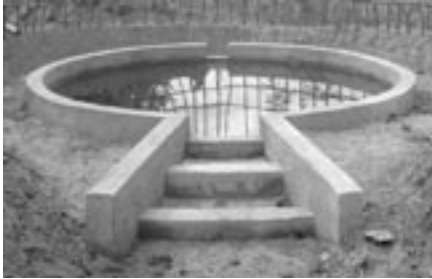
Run off rainwater harvesting tank
