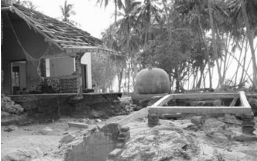
Tsunami damage in Sri Lanka
