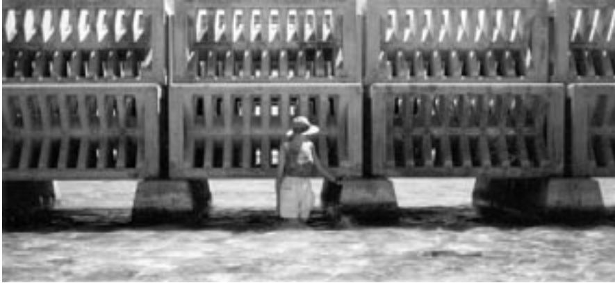
Concrete coastal protection device, Raratonga International Airport
