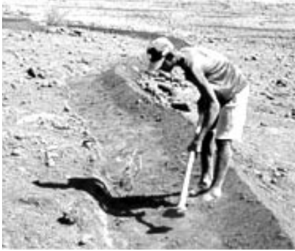
Creating a contour ridge to trap water run-off, Cape Verde
