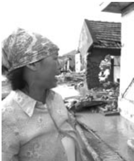
Storm damage in Vietnam
