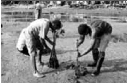
From top to bottom: villagers planting vetiver grass at Buretu; new roof-fed communal water tanks at Bavu; replanting mangroves at Navukailagi
