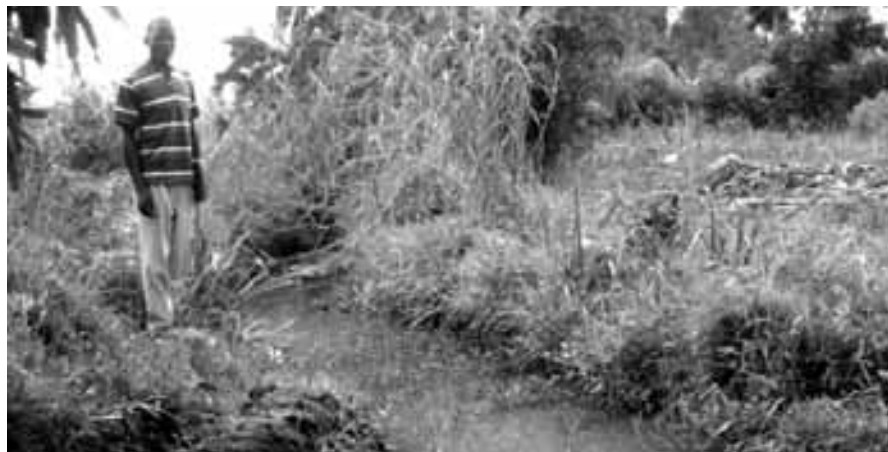
A community leader shows the expanded drainage canals
